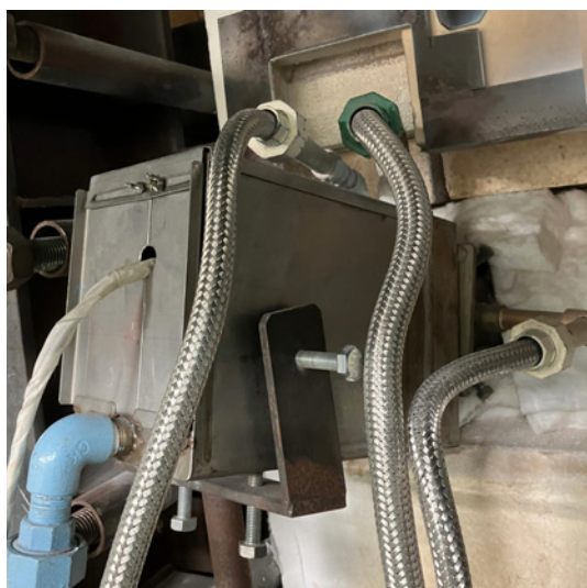
Installation of ITV equipment
