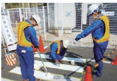
Painting zebra crossing on plant premises
